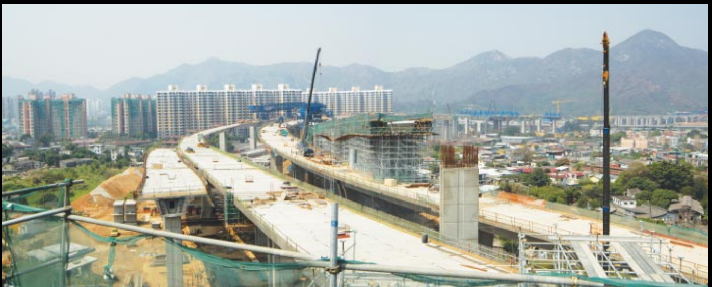
The overview of the east-bound section of Lam Tei Interchange from the falsework platform erected for the construction of the cross road along Yuen Long Highway
