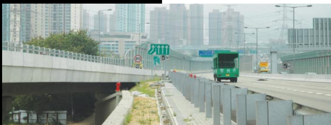
The slip road inlet entering Yuen Long Highway from Lam Tei Interchange heading to Fu Tei direction. The extra lane and the road shoulder at the left side of highway are newly formed and re-aligned using land-filling supported by retaining structure during the widening process
