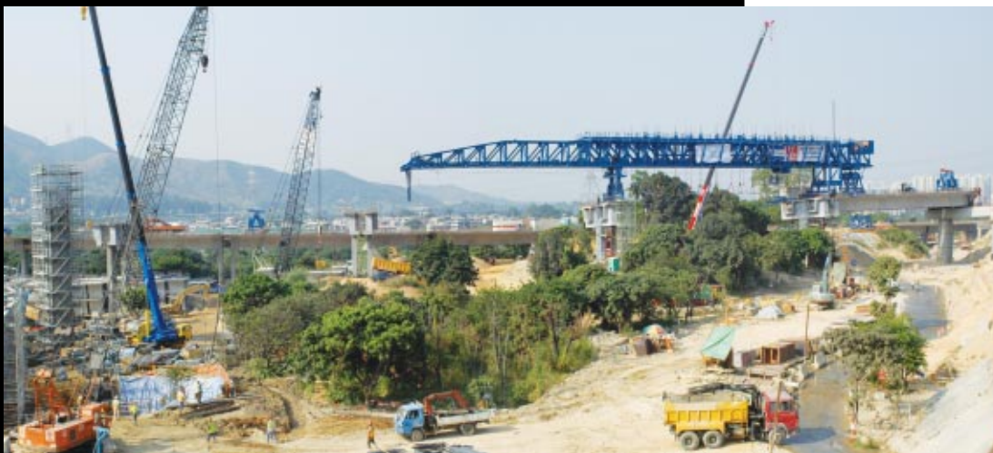
A set of launching gantry used to lift and erect the precast segments for the construction of the viaduct. The section of 800 m-long viaduct as shown in this photo is the east-bound carriageway finally joins the Route 3 via Yuen Long Highway
