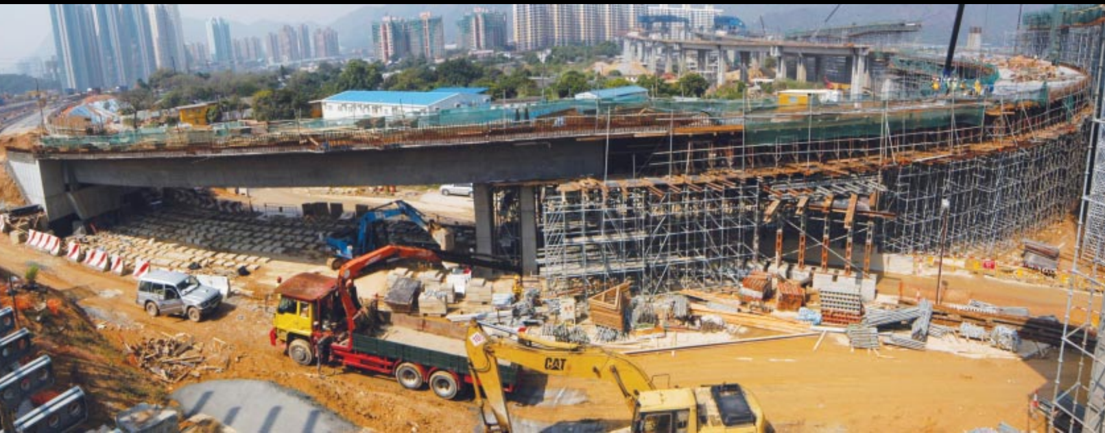
The construction of the slip road entering from east-bound direction of Yuen Long Highway (left) into Deep Bay Link (right). The buildings on the background are located in the area of Fu Tei, Siu Hong and Lam Tei as positioned from the left to the centre of photo
