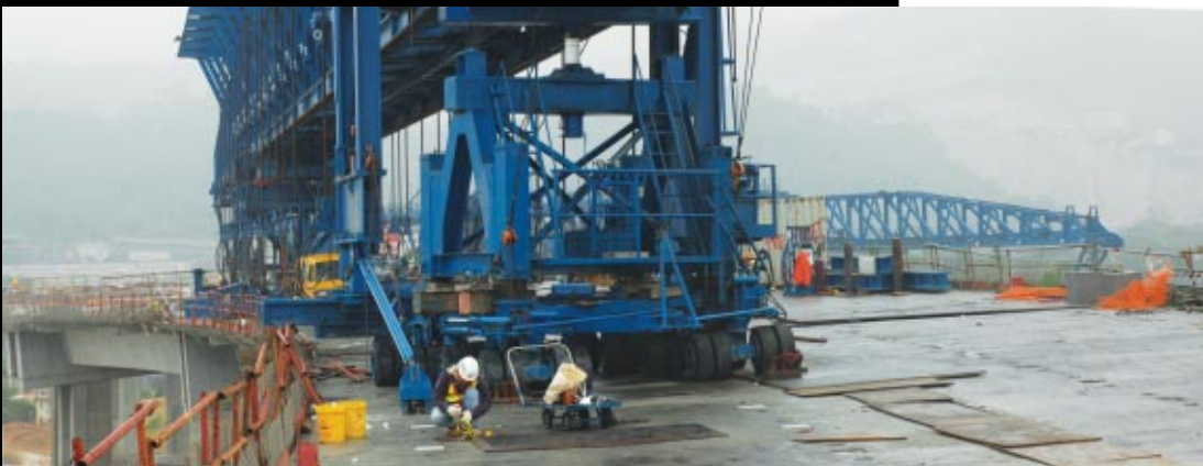
View on the deck level stationed with a launching gantry preparing for the repositioning to a new location for the construction of a new viaduct section
