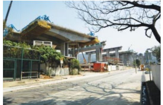
Rows of portal frames running across Castle Peak Road (outside photo on left) before joining into Lam Tei Interchange. The maximum width of the carriageway at this section is totally 8 lanes, with dual 3-lane entering into the interchange and dual single-lane provisioned for a future outlet leading into the existing Castle Peak Road
