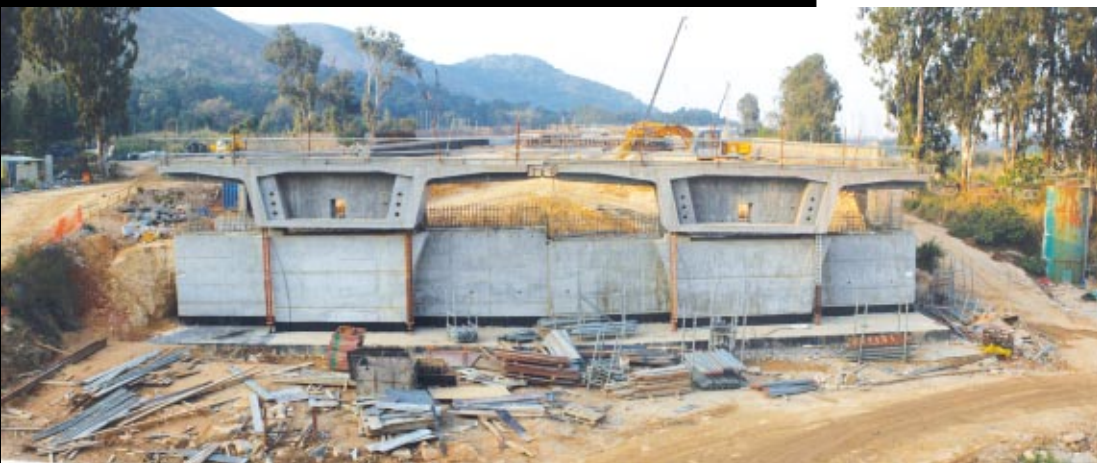
There are a few sections of Deep Bay Link (Northern Section) constructed at-grade. Various forms of abutment structure would be provided to receive the carriageway from elevated to at-grade position. This photo shows a section of abutment structure at Ha Tsuen (厦村) with the head segment already in place
