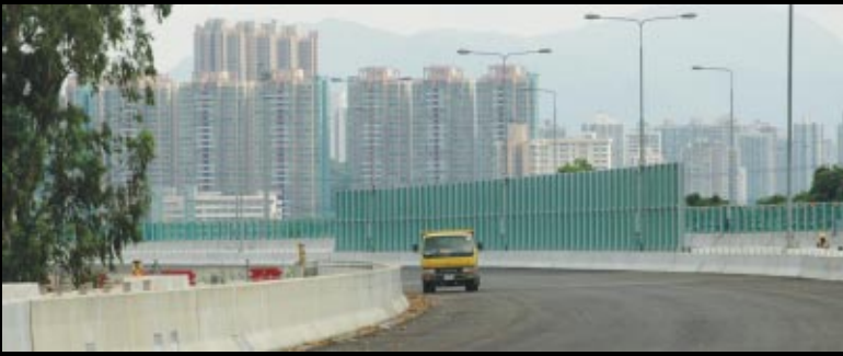
Deck view near the adjoining link between the Northern and Southern Section with the noise screen erected before the handing over. The high-rise buildings forming the background are the residential development in Lam Tei area
