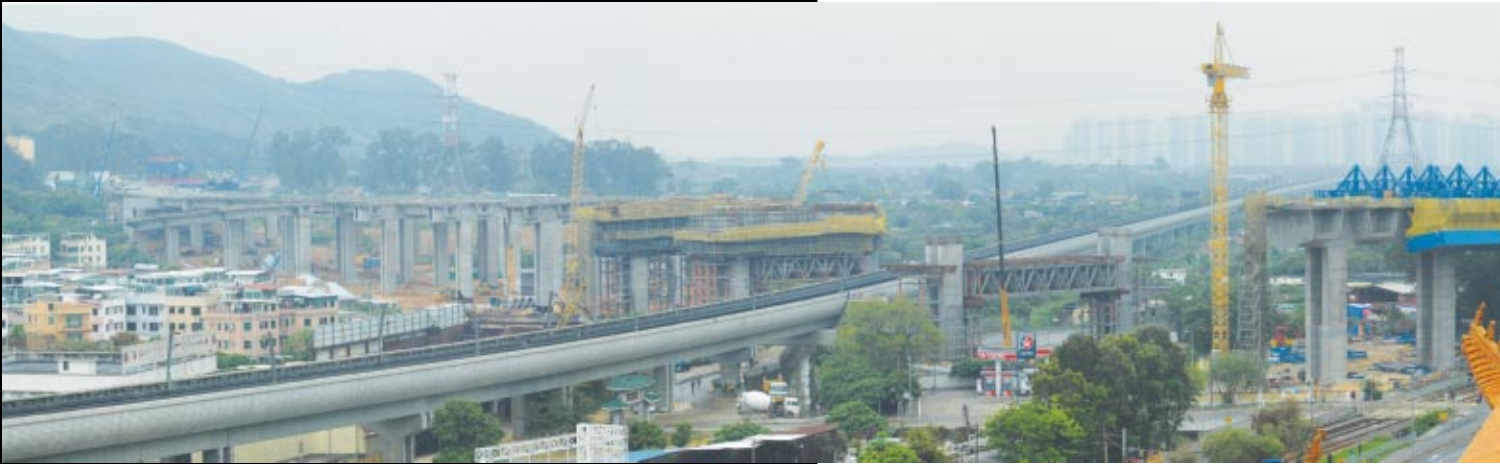
Panoramic view seeing the viaduct approaching the elevated track of West Rail from Yick Yuen Chuen and Ching Tsuen Wai before the crossing over. The portal frame on the right side is the joining section between the Northern and Southern Sections of Deep Bay Link
