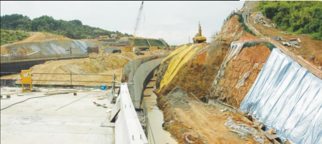
Close up of the slope cutting and the carriageway approaching the at-grade section. Backfilling to the abutment side and slope treatment with landscaping provision would be done at a later stage
