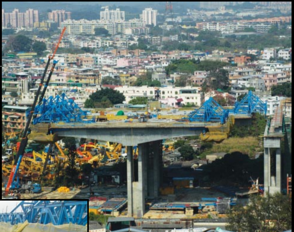
Close up of a section of the viaduct constructed in balanced-cantilever arrangement using sets of girder-mounted traveling formwork on both ends. The village houses around Yick Yuen Chuen forms an impacting background showing the fragile nature of the project environment
