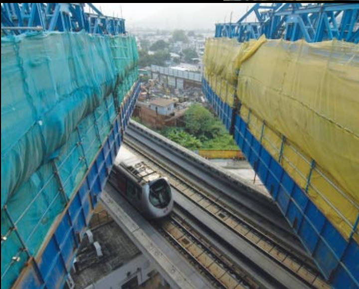
From the viaduct viewing downward seeing a train rushing through the elevated track of West Rail. The gantry in blue on each side is the traveling formwork system used to cast the box-section deck of the viaduct in-situ
