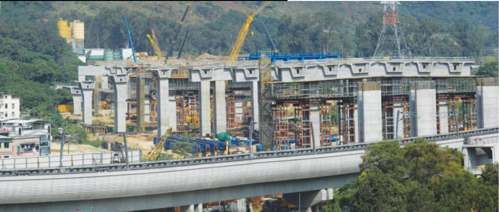
Rows of portal frames approaching the track of West Rail as viewed in early 2005
