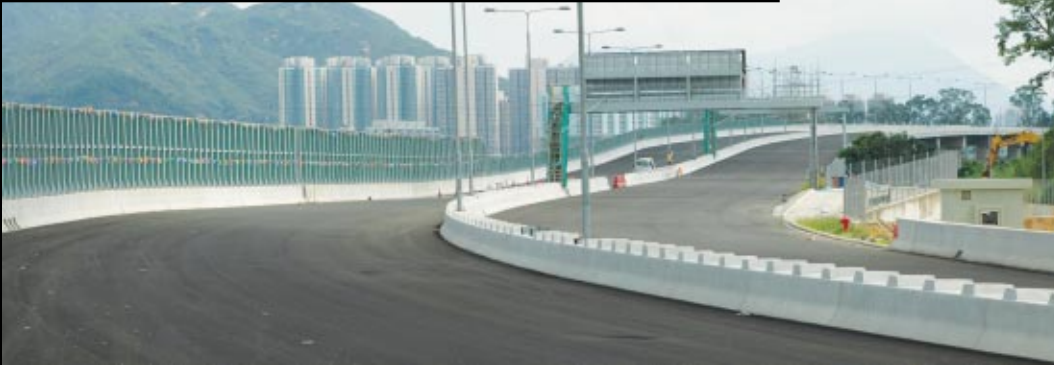
Deck view near the adjoining link between the Northern and Southern Section with the noise screen erected before the handing over. The high-rise buildings forming the background are the residential development in Lam Tei area
