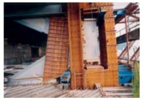
Photo 34: Close-up of the column/outrigger joint with the provision of a slot to control differential shortening
