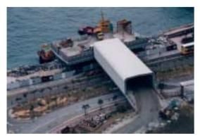
Photo 44: Temporary pier set-up along the seawall outside the site for dumping purposes
