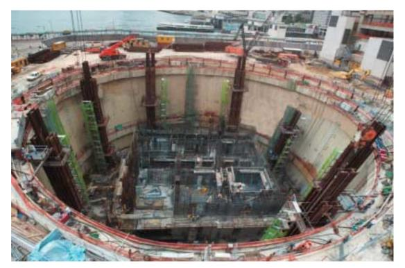
Photo 7: A view into the cofferdam with the core wall and mega-columns in position close to ground level
