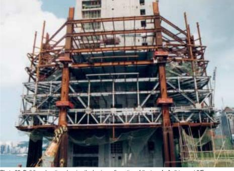
Photo 25: Building elevation showing the basic configuration of the transfer/belt truss at 6/F
