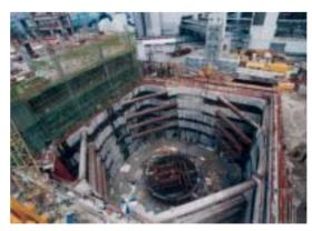
Photo 53: 42 m X 42 m cofferdam formed on the western part of the site for the construction of a vehicular ramp as access into the carpark in the future basement
