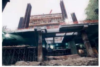
Photo 38: Commencement of the top-down basement. The work arrangement with steel stanchions supporting the ground floor slab and the basement excavation/construction underneath can clearly be seen
