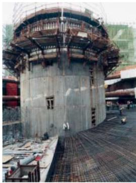
Photo 57: A detailed look at the gang-form system for the construction of the circular core and the steel bar fixings before the concreting of the ramp
