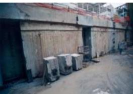
Photo 45: Double-bit arrangement to construct the basement floors. An intermediate basement slab, positioned where the excavating machine was located, was being cast in an advanced phase and also served as a separating plate where the upper slab could be constructed while allowing excavation below to safely proceed at the same time
