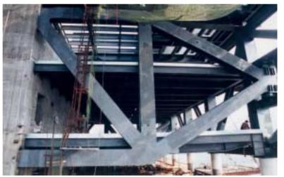
Photo 36: The arrangement of the outrigger system used at Cheung Kong Center (at 59/F)
