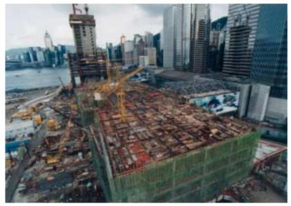
Photo 50: An overview of the podium structure before topping-out
