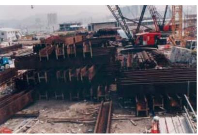
Photo 10: Steel sections stacked on the site for forming the mega-columns
