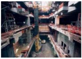
Photo 41: Looking into the muck-out opening with the excavation arrangement clearly seen
