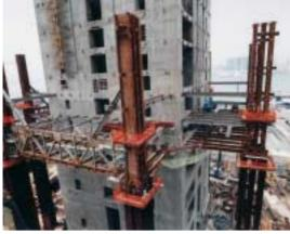
Photo 8: Forming the transfer truss at 6/F at its early stage. Also note the size reduction of the mega-columns at this level
