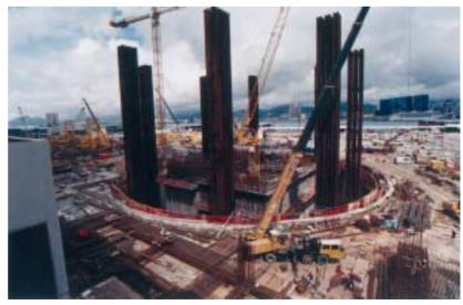
Photo 11: Work stations around the sides of the cofferdam on ground level, forming an important base to serve construction activities inside the cofferdam
