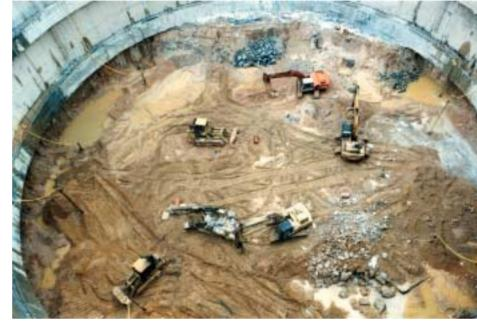
Photo 3: Excavation in progress at the formation level of the 61 m diameter cofferdam
