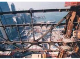
Photo 26: Configuration of the 32/F belt truss before the erection of the floor beams and floor plates
