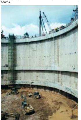
Photo 4: The 61 m diameter cofferdam formed by 1.5 m thick diaphragm wall panels was strengthened by RC ring beams
