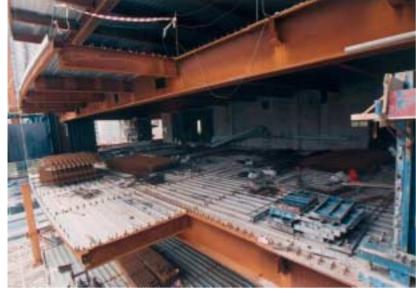
Photo 20: A 24 m edge beam spanning between the mega-columns at the lower section of the tower. The beam sections were gradually reduced in size for higher levels
