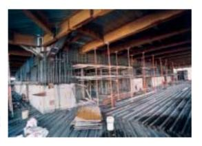
Photos 32a & 32b: Encasing of the anchor frame and reinstatement of the core wall
