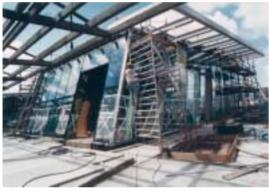
Photo 52b: A close up look at one of the three glass hoods on the roof deck during its installation
