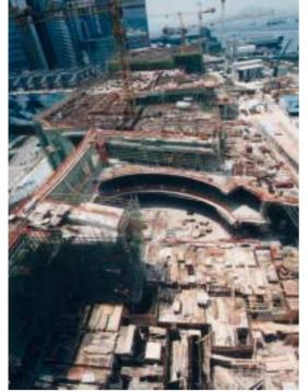
Photo 51b: A close up look at the podium structure which used rather traditional timber formwork in construction
