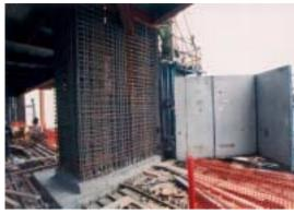
Photo 24a: The climb form in position ready for encasing
