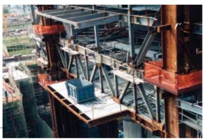
Photo 9: Detail of the south elevation of the transfer truss at 6/F
