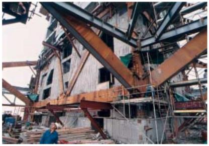
Photo 30: Installation of the outrigger system at 32/F — anchor frame being installed onto the core wall recess. The frame was encased in reinforced concrete at a later stage, after completion of the floor system
