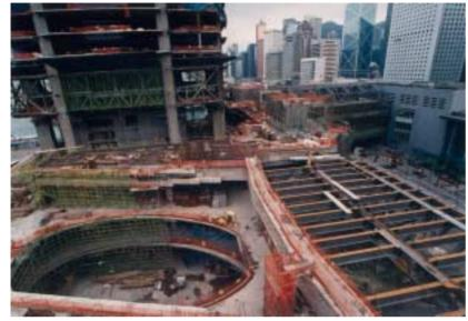
Photo 48: The forming of a 25 m-span oval-shaped atrium with 20 m headroom inside the podium structure
