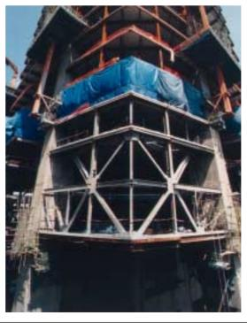
Photo 17: A view of the climb form at a building corner when it was in the released position ready for lifting to the next working level
