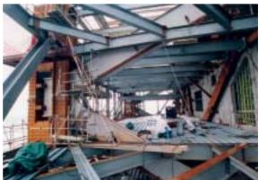
Photo 27: Part-detail of the outrigger/belt truss system at 54/F
