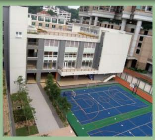
he project comprises the construction of a 6-storey 24-classroom school building consisting of a classroom block and an assembly hall block overall T-shaped on plan together with associated facilities.
