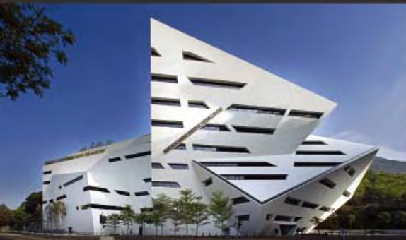
Run Run Shaw Creative Media Centre, City University of HK, HK (Studio Daniel Libeskind with Leigh & Orange Ltd.)
