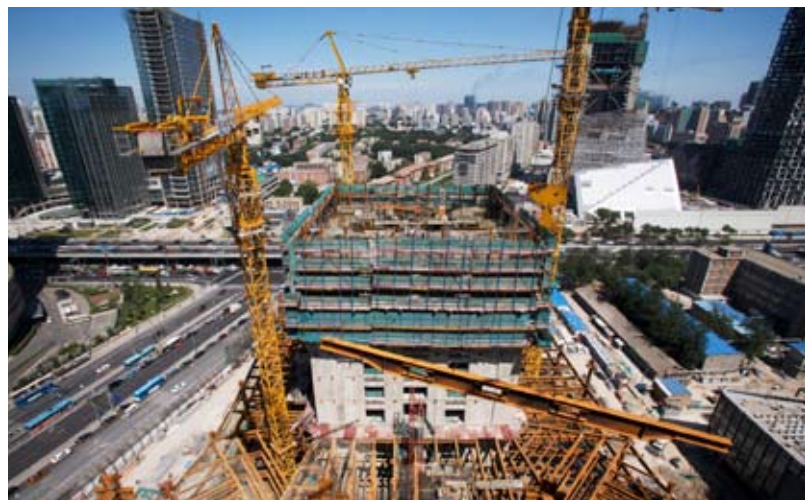
Hydraulic self climbing formwork and prefabricated structural steel
