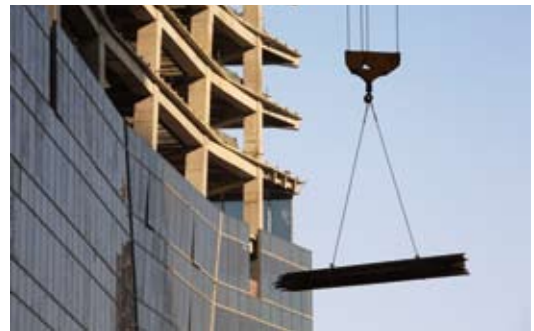
Typical floors and unitized curtain wall under construction
