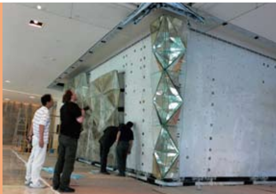
Installation of Crystal Wall under artist Michael Hammers' supervision
