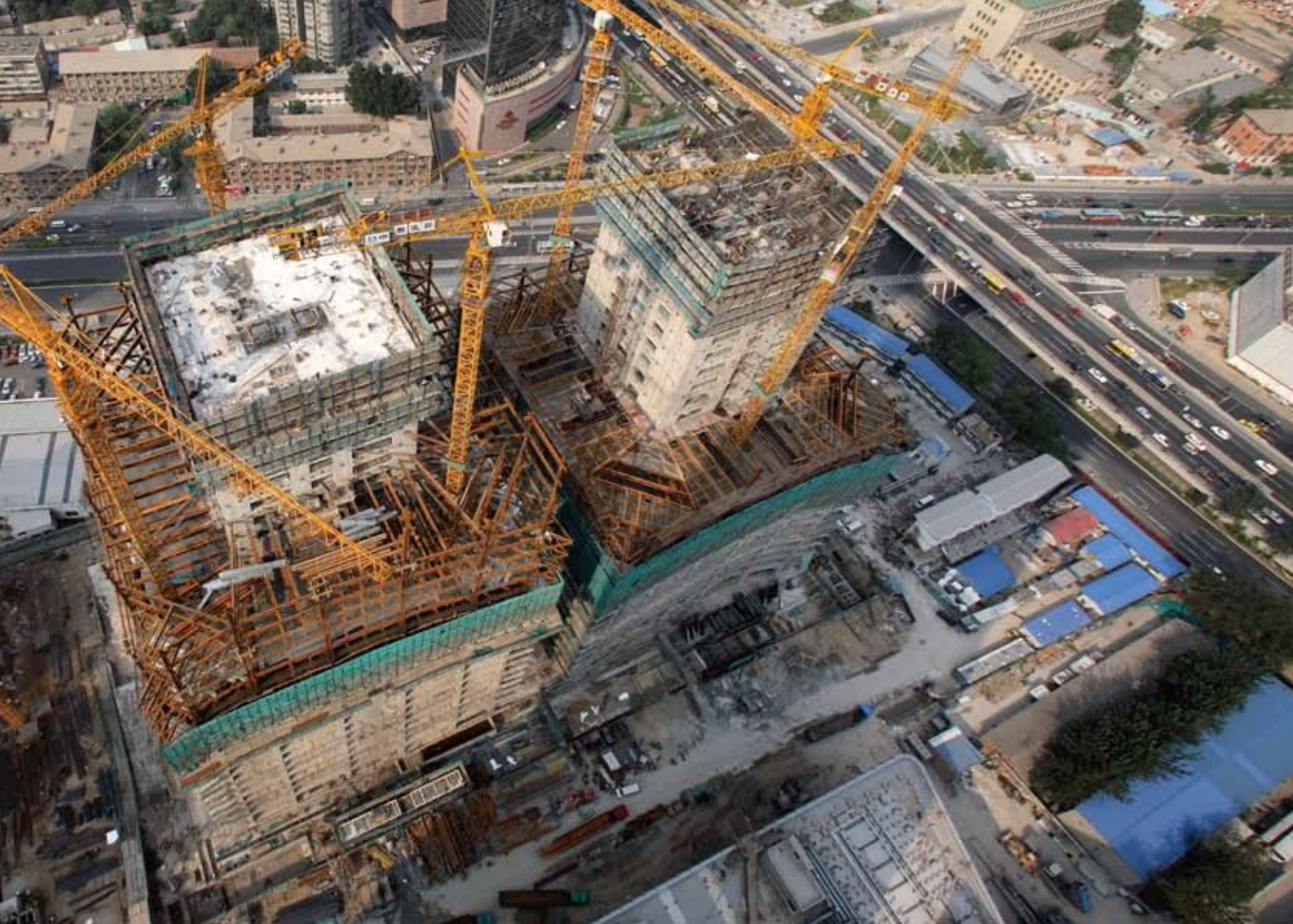
Areal view of site showing mechanized construction methods
