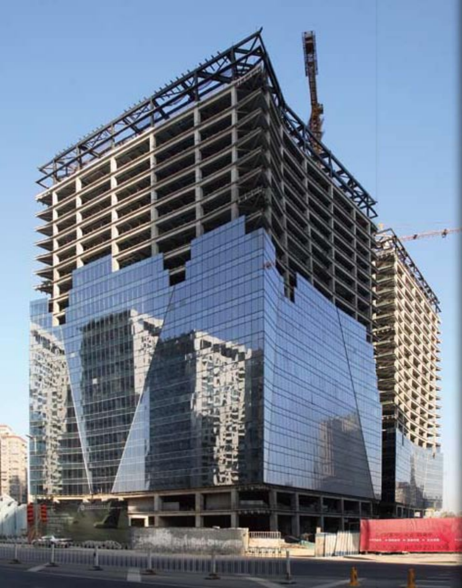
Installation of modular double glazed, low-e, argon filled curtain wall system
