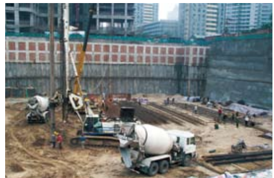
Basement and piling under construction in shoring free excavation
