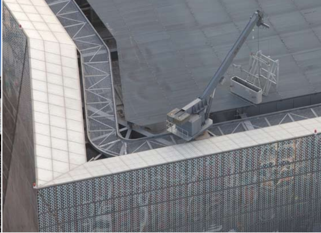
Building Maintenance Unit (BMU) at roof top (two on each tower)
