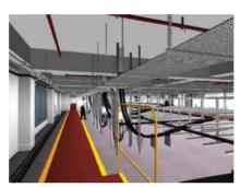
Cable basement with defined trays for power cables and demarcated escape route
