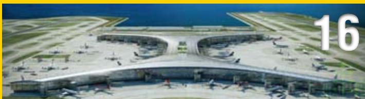
3RS development, Hong Kong International Airport
