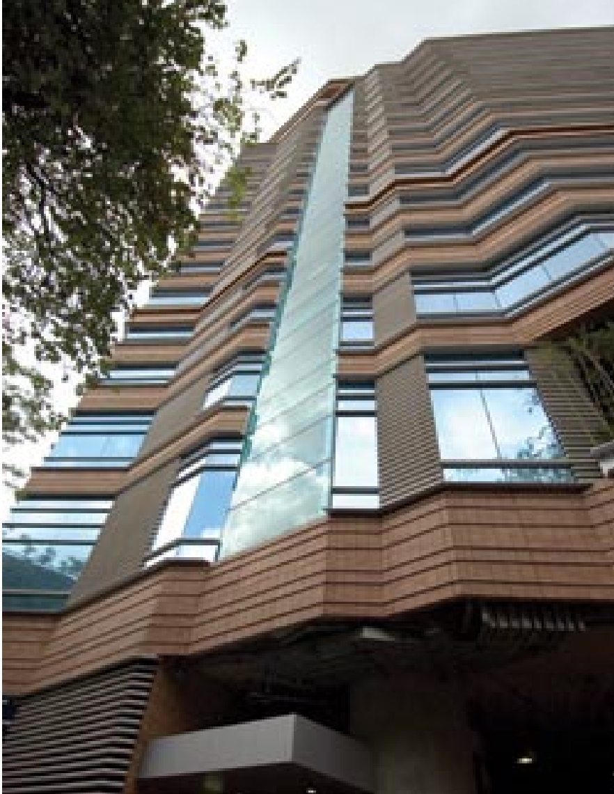
14 Lee Shau Kee Building, The Hong Kong Polytechnic University
